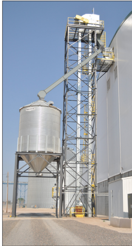
Closeup view of the flat storage receiving and loadout system at Kimball, NE with GSI InterSystems leg and Brock surge tank. Ground-level photos by Ed Zdrojewski.
