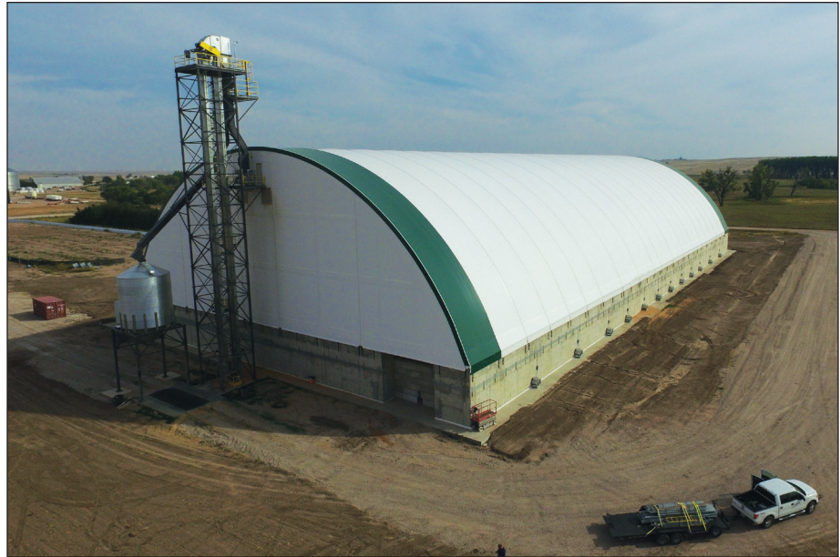
New 2-million-bushel flat storage hoop building at Frenchman Valley Farmers Cooperative in Chappell, NE. Drone aerial photos courtesy of Macon Construction.
