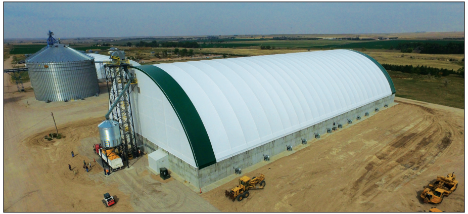
New 2-million-bushel hoop building at Kimball, NE.
