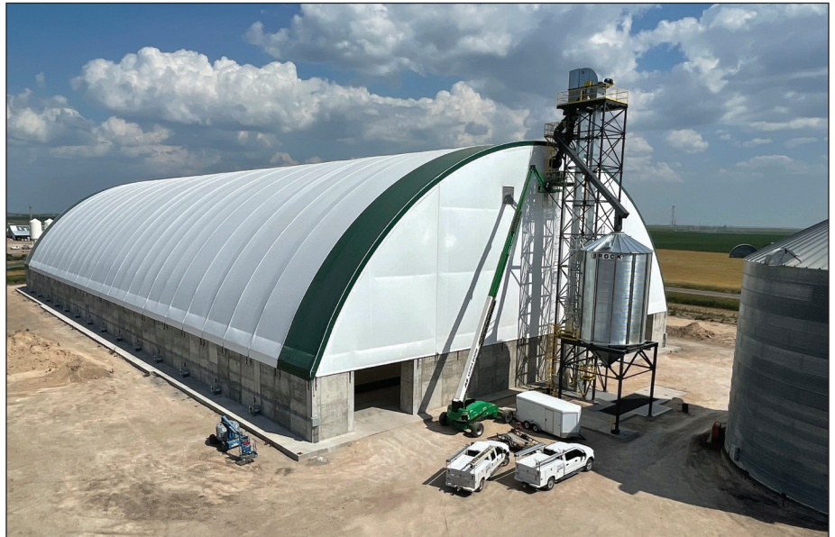
Another 2-million-bushel flat storage nearing completion at Grant, NE in July 2021.
