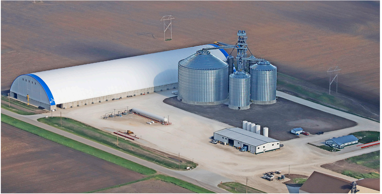
Landus' new 5.54-million-bushel elevator near Mitchellville, IA features a 3.9-million-bushel Macon Construction hoop flat storage building and three Sukup steel tanks. Aerial photo by JH Photography, Spencer, IA.
