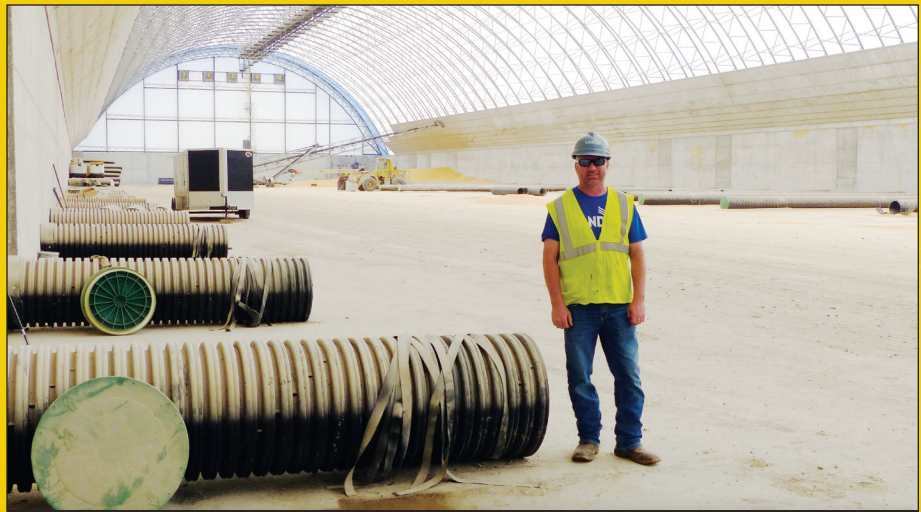
Landus Hub Lead Jason Lemmert inside the Macon Construction 180-foot-x-660-foot fabric-covered hoop flat storage building.
